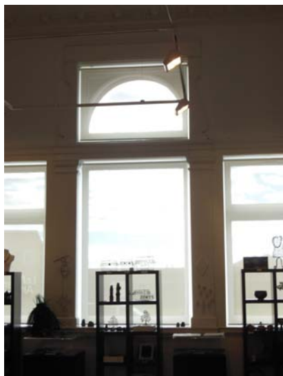
Looking north at window mullions
