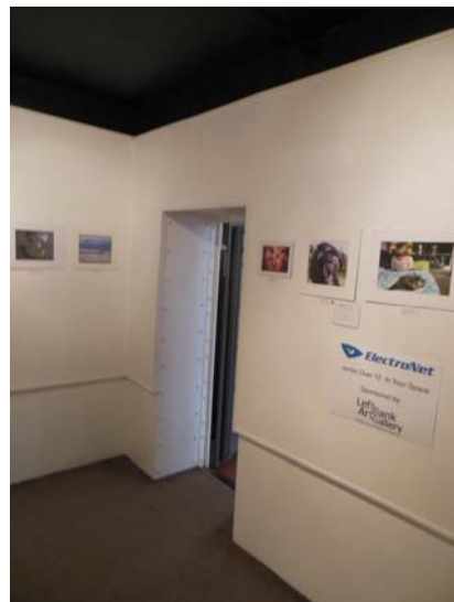
Inside concrete strong room
